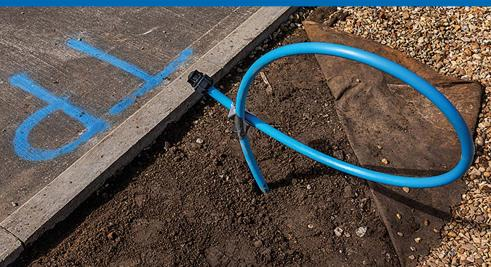
A minimum 2 metres of pipework exposed and the end of your tailpipe sealed with a compression cap coming up from ground level on the edge of your boundary and/ or at the agreed connection point. This will be marked by us with a blue 'TP'. We will endeavour to be at least 2 metres clear from any street furniture i.e. lamppost, telegraph pole, etc.
