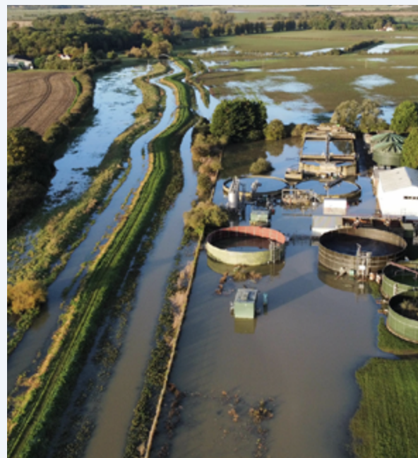
Anwick Water Recycling Centre under water. Image credit: Paul Barham, Maintenance Support Technician.
