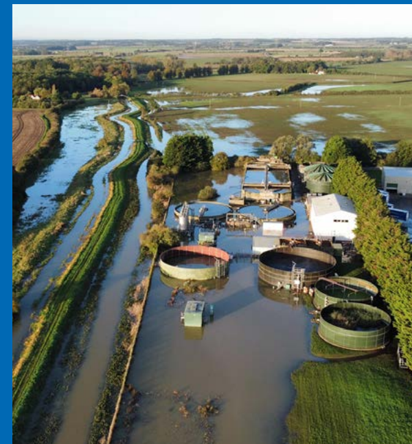
Anwick Water Recycling Centre under water. Image credit: Paul Barham, Maintenance Support Technician.
